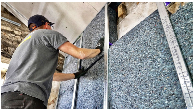
Building insulation panels made by Buitex from post-consumer waste
